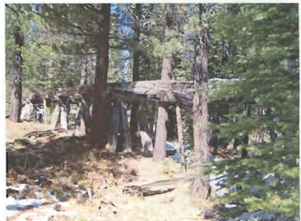
Independence Creek trestle (Hobart Mills).
