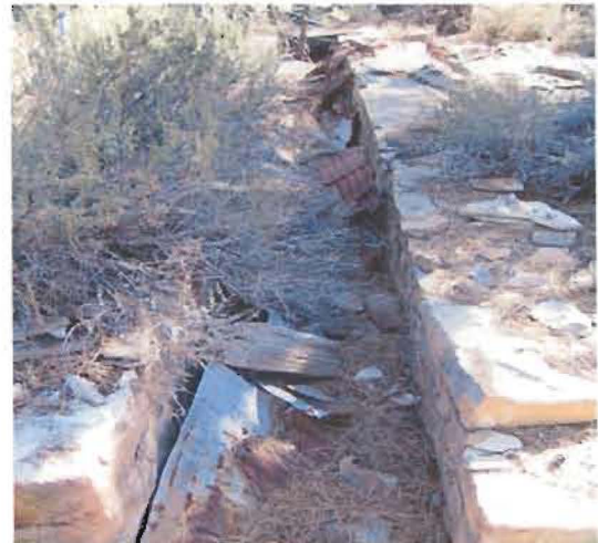
Engine house work pit at Hobart Mills. There was an eight stall round house at this site.
